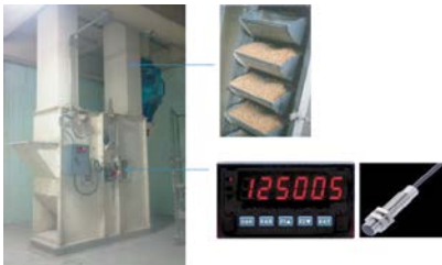
Control Speed Bucket Elevator ติด Proximity and Counter
